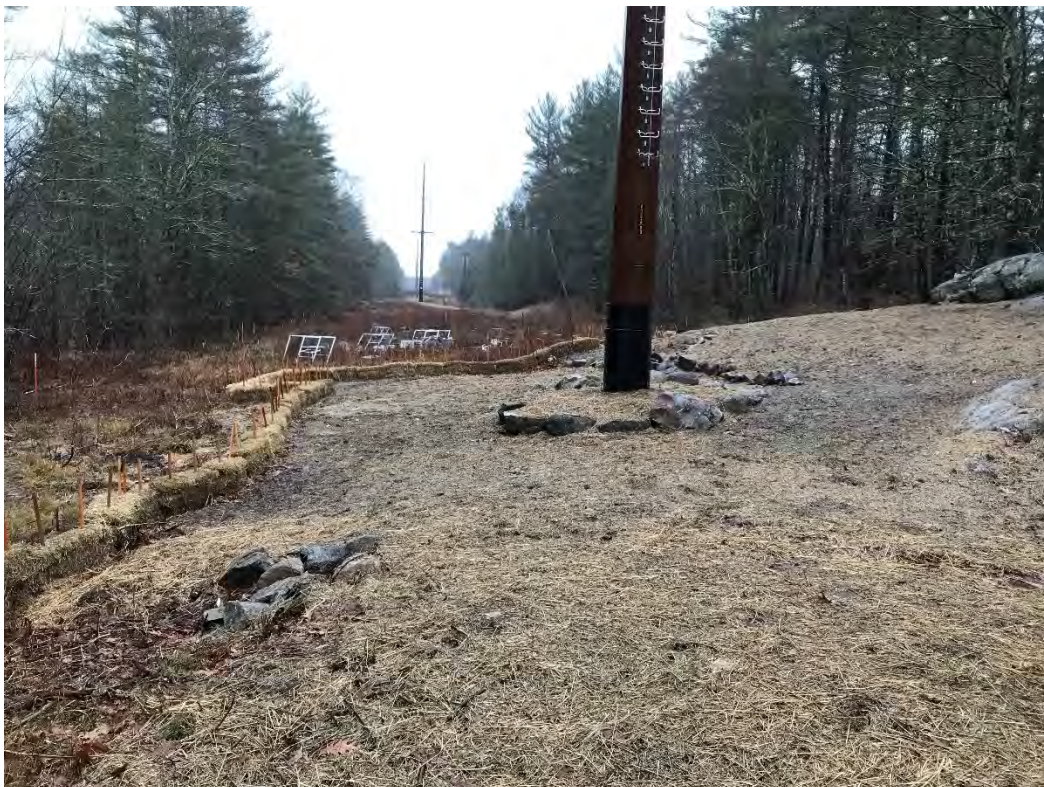
Fig 4: Str. 89 work area. Viewing southeast. (01-16-21)
