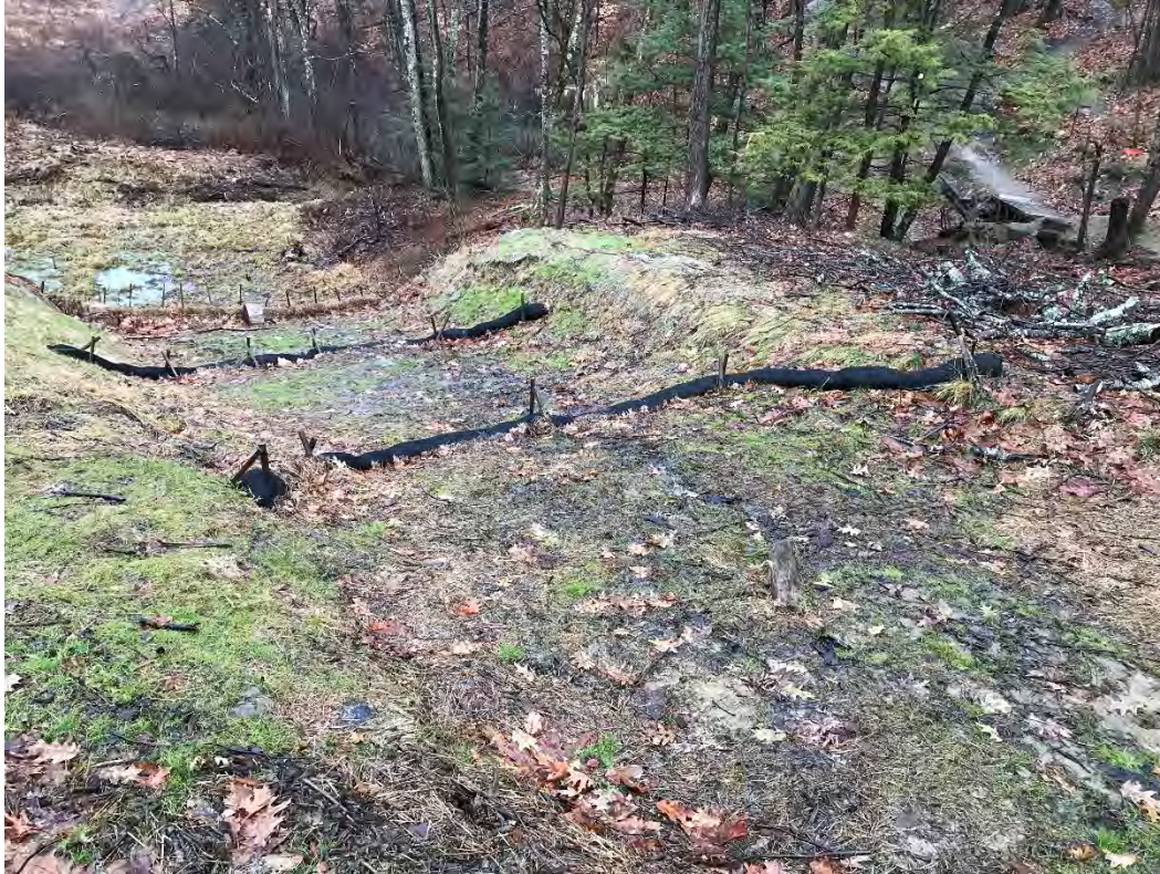
Fig 7: Lower portion of slope between Strs. 28 and 29. Viewing northeast. (01-16-21)
