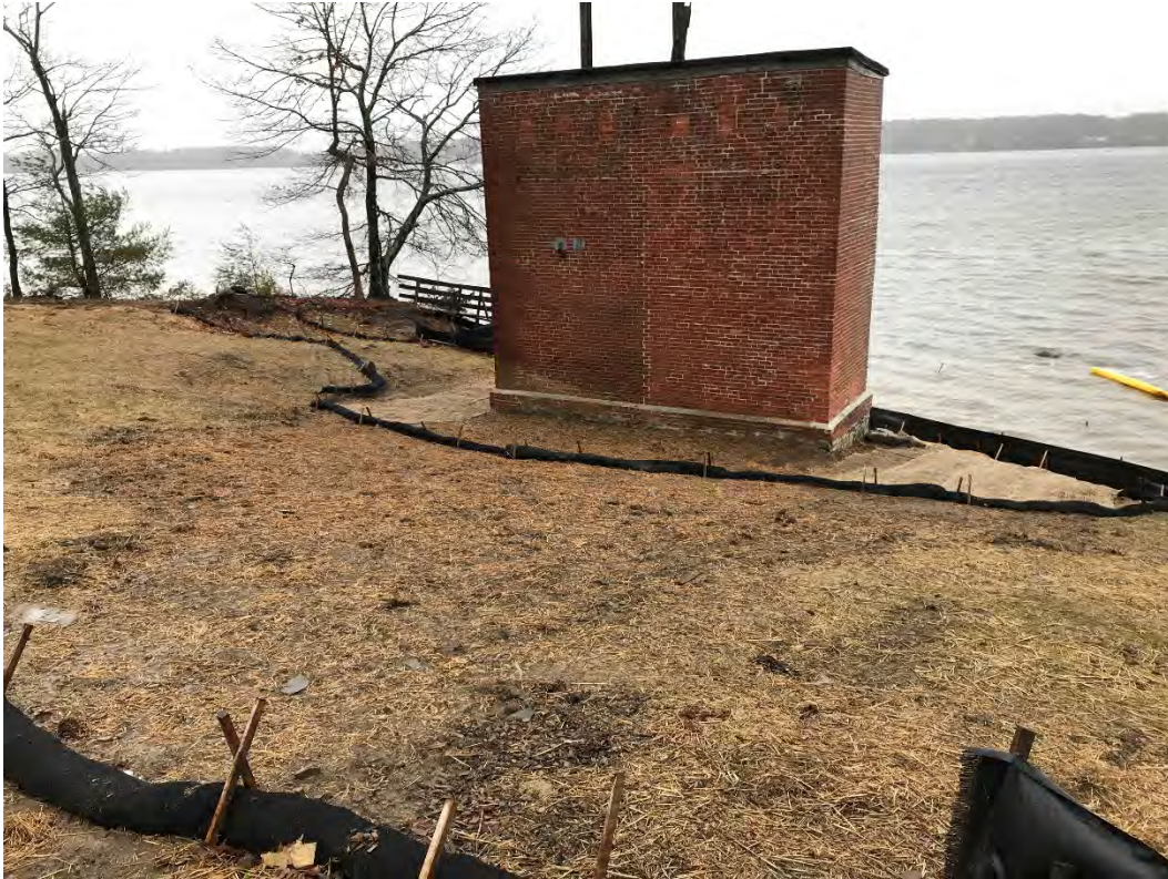
Fig 1: Slope leading down to cable house and salt marsh restoration at the Eversource property/west side of the bay. Viewing northeast. (01-16-21)
