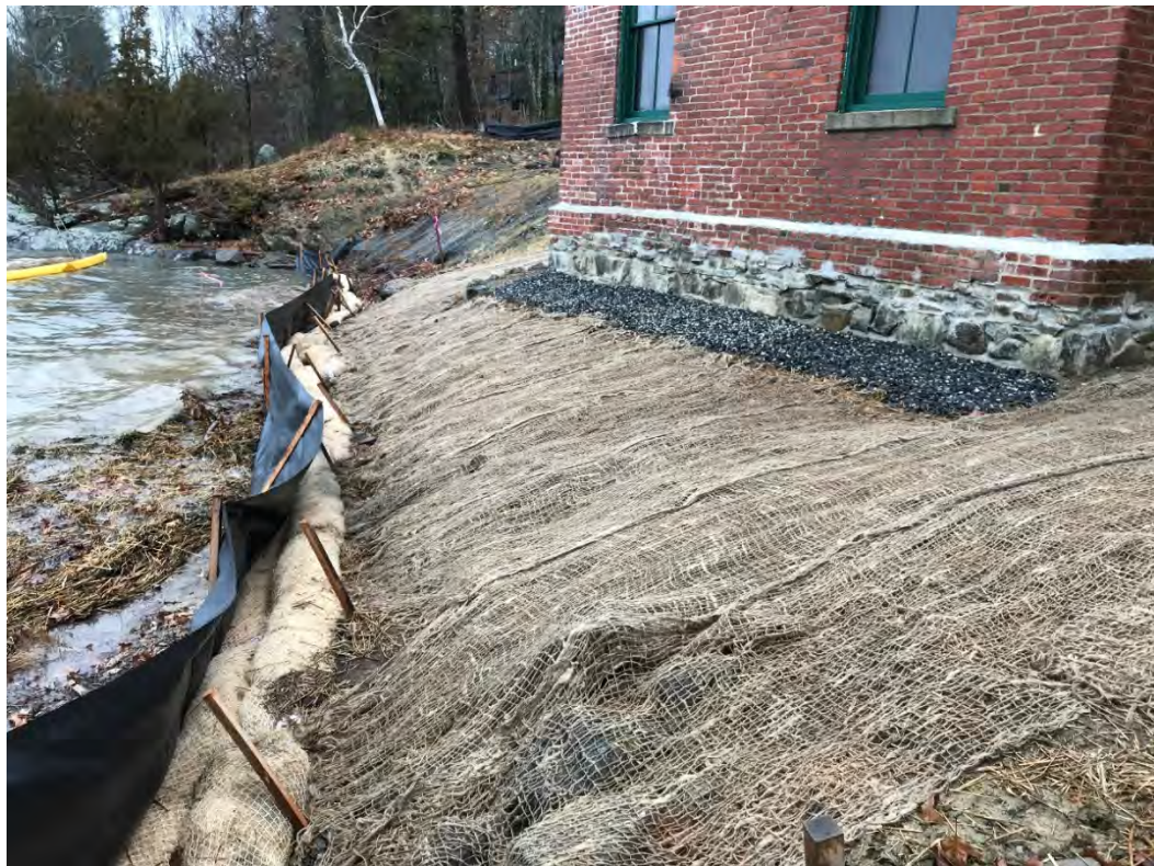
Fig 2: Stabilized slope between the cable house and salt marsh restoration at the Eversource property/west side of the bay. Viewing south. (01-16-21)
