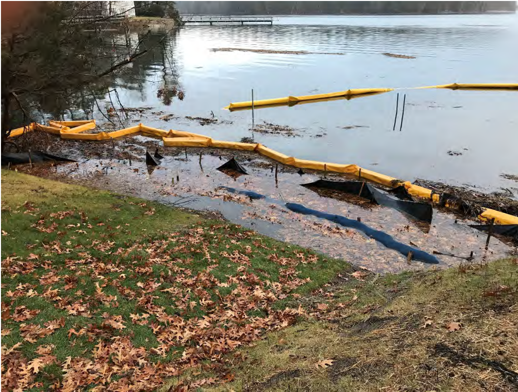
Fig 11: Toe of the slope at Gundalow Landing/east side of the bay. Viewing south. (01-16-21)
