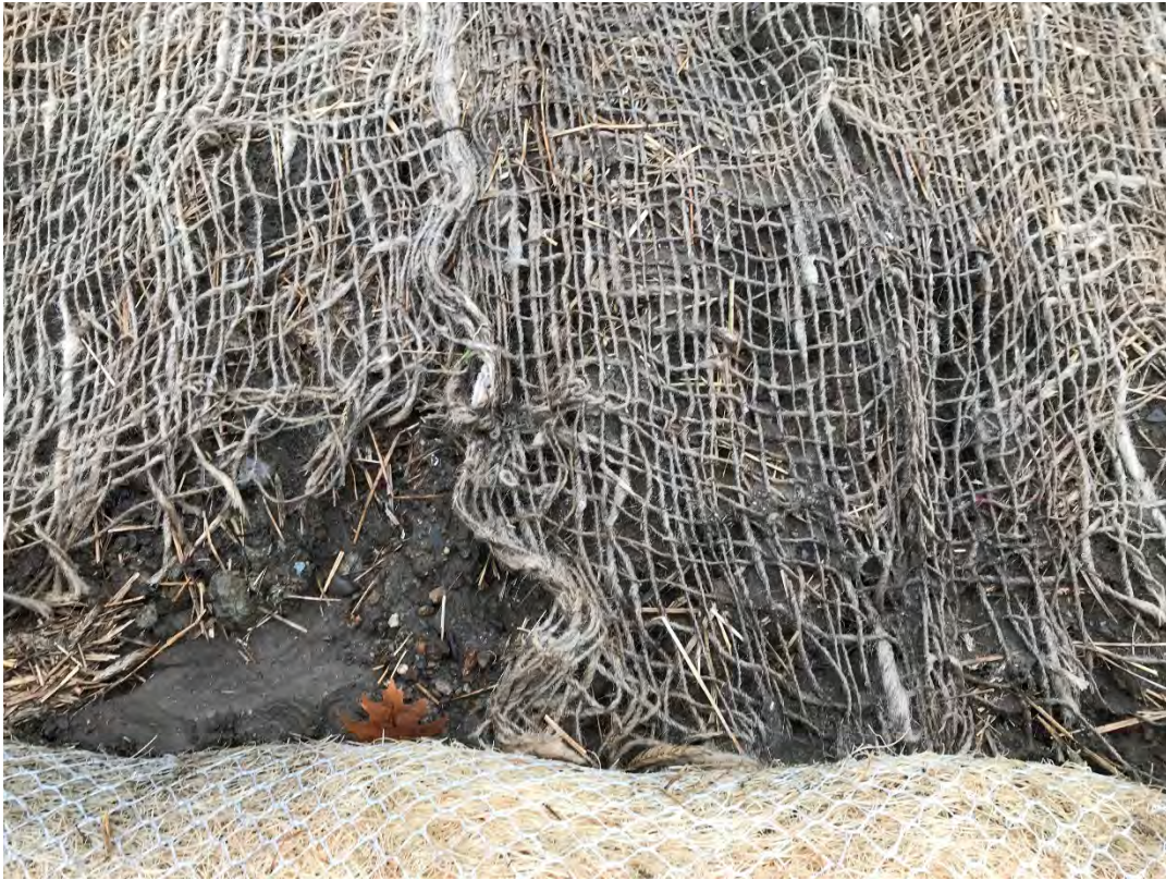
Fig 3: Minor rills and sedimentation on the slope above the salt marsh at the Eversource property/west side of the bay. Viewing west. (01-16-21)
